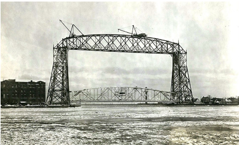
Construction to convert the Aerial Ferry Bridge to the Aerial Lift Bridge in 1929. Image courtesy of Kathryn A. Martin Library Archives and Special Collections at UMD
