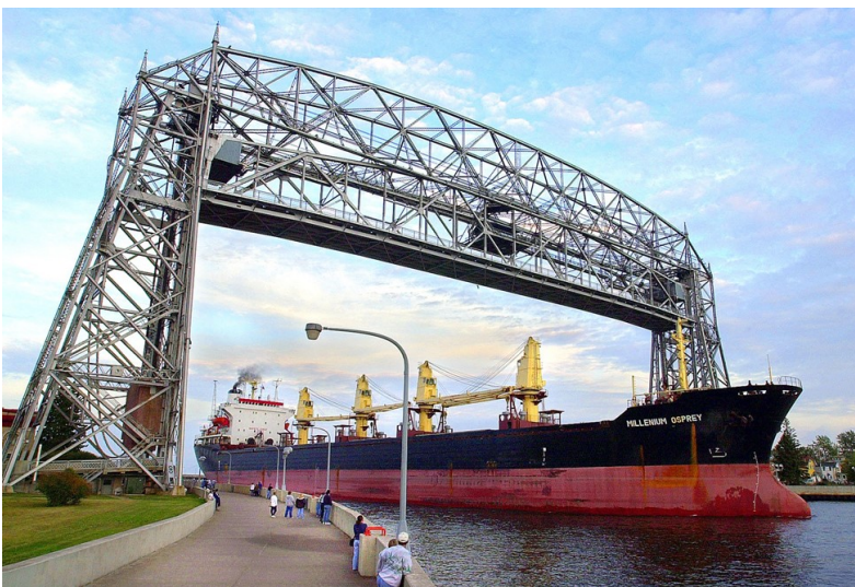
The oceangoing vessel Millenium Osprey passes under the Aerial Lift Bridge in September 2001. Photo by Justin Hayworth, courtesy Duluth NewsTribune
